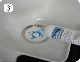
Pour about **30 oz. of water** over the Drain Insert. Then slowly pour the **entire contents of the Odor Barrier** onto the Drain Insert. Wipe clean. The ZeroFlush Urinal is now ready for use.
