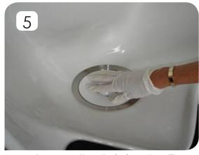
Press down on the drain insert until you feel and hear a slight popping sound. The insert must be tight.
